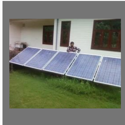
Off Grid Solar Power
