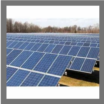
Solar PV Power Plant
