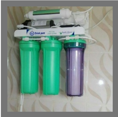
Water Purifier Installation Services
