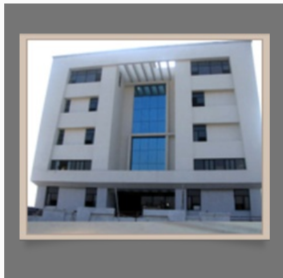
Structure Glazing : Structural glazing
