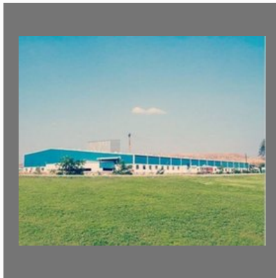
Commercial Building Construction Services
