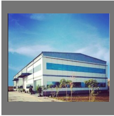
Industrial Building Construction Services
