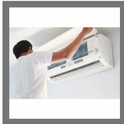
Split Ac Installation
