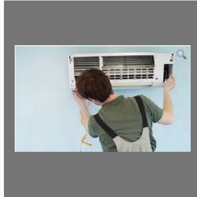
Split Ac Installation Services
