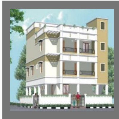
1 Bhk Apartment Construction
