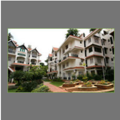
Mangalya Residences Construction Service
