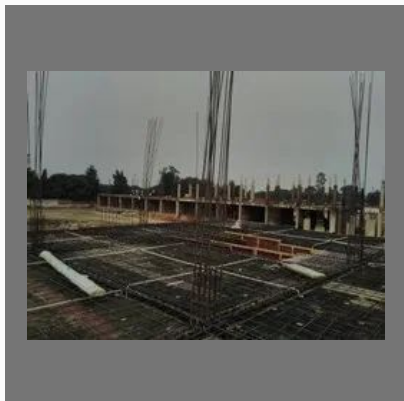
Construction Services For School Building
