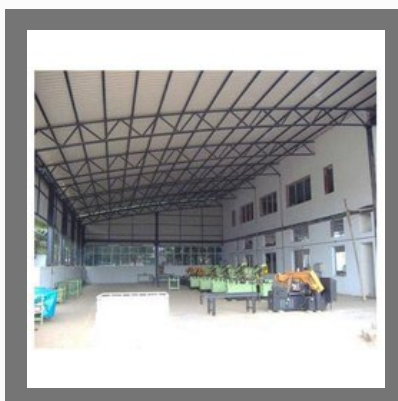
Industrial Prefabricated Factory Shed
