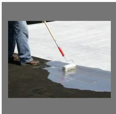
Roof Waterproofing Services
