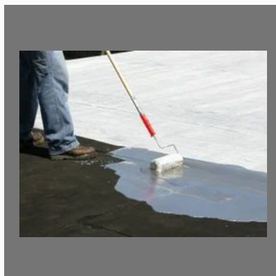
Roof Waterproofing Treatment
