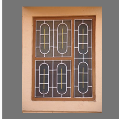
Iron Windows Grill
