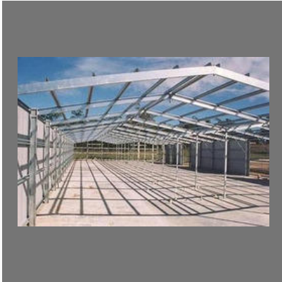
Heavy Industrial Shed
