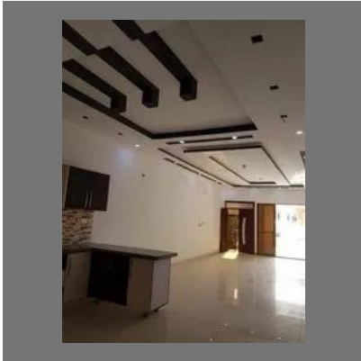
Gypsum False Ceiling
