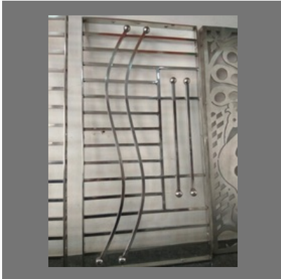
Steel Window Grill
