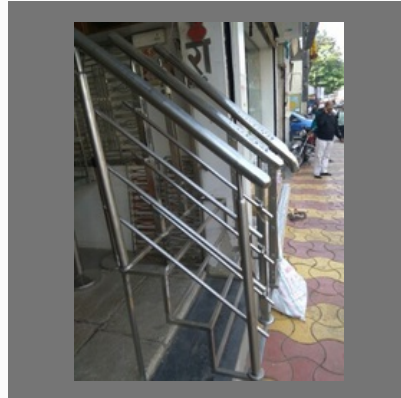
SS Steel Railing
