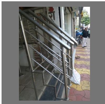
SS Steel Railing
