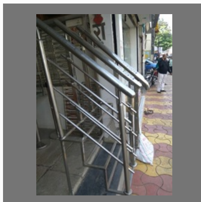
SS Steel Railing
