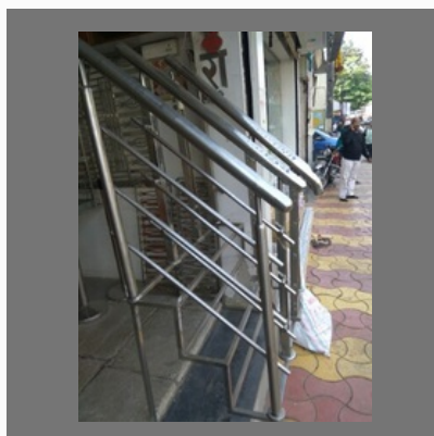
SS Steel Railing
