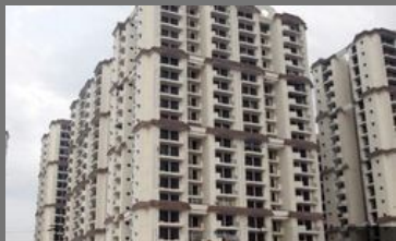
Residential Apartments Construction
