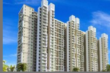
Residential Building Construction
