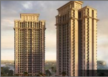
Building Construction Work
