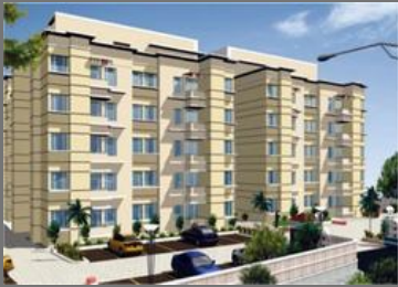
5BHK Flat Construction Services
