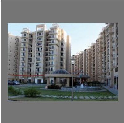
Commercial Building Construction Services
