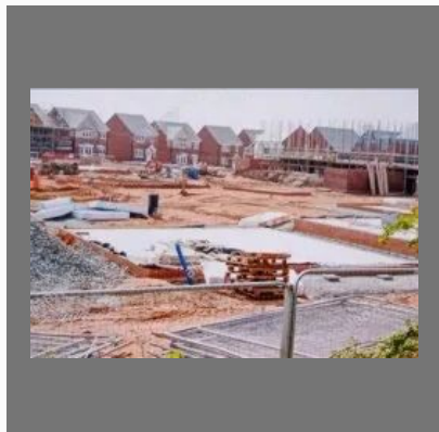
Construction Work Of Site
