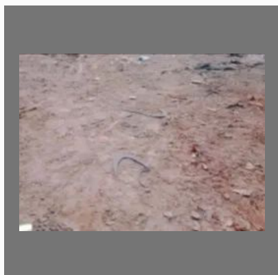
Road Side Construction
