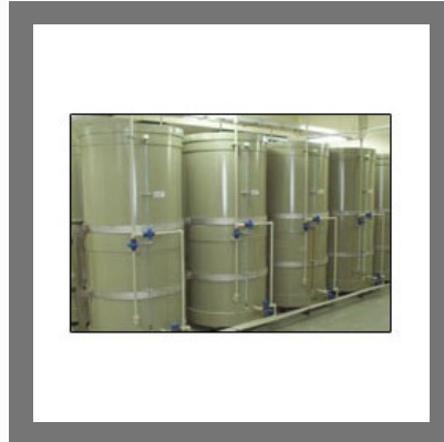
Oil Storage Tank
