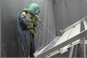
Shot Blasting Work
