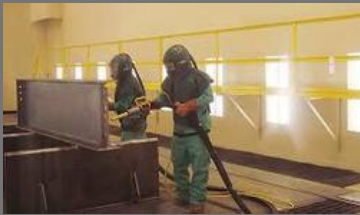
Sand Blasting Work
