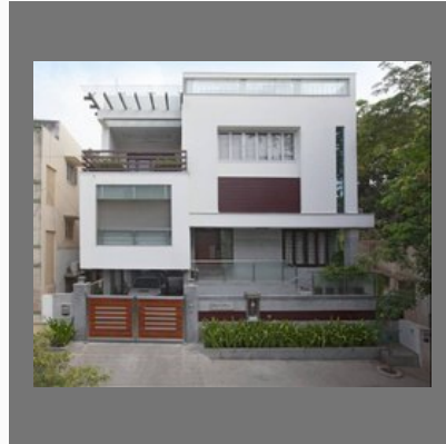
Residential Construction Service
