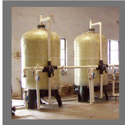
ACTIVATED CARBON FILTER
