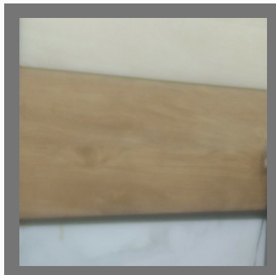
Wooden Floor Tiles
