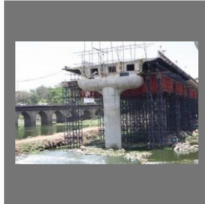
Pier & Girder Shuttering
