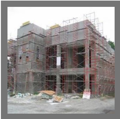
Construction Scaffolding Rentals
