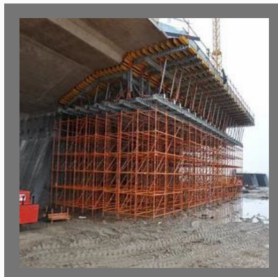
Bridge Formwork And Staging
