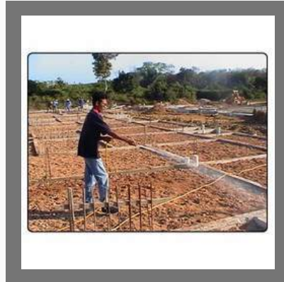
Pre Construction Anti Termite Treatment Services
