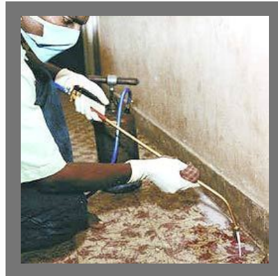
Anti Termite Treatment For Floor
