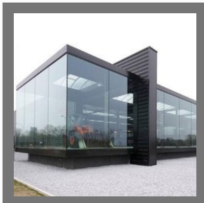
Office Structural Glazing
