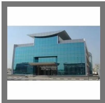
Commercial Glazing Building
