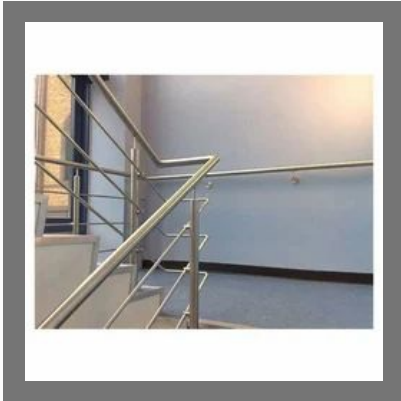
SS Hand Railing
