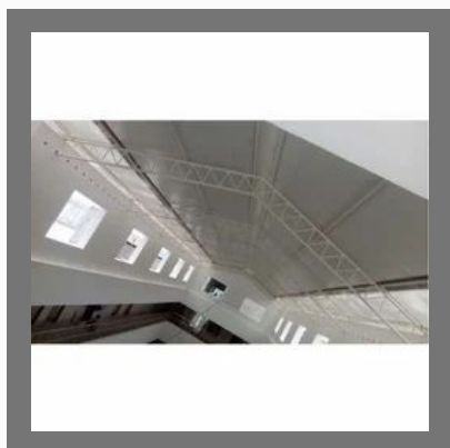
Warehouse Roof Truss
