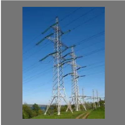
Transmission Line Towers
