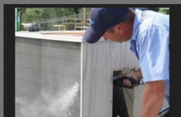
AHU Cleaning Services
