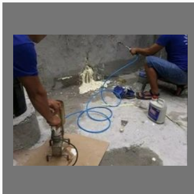
Waterproofing Pressure Grouting in madhya pradesh
