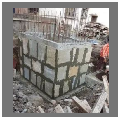
Basement Waterproofing Services in madhya pradesh
