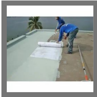
Industrial Roof Waterproofing In Indore
