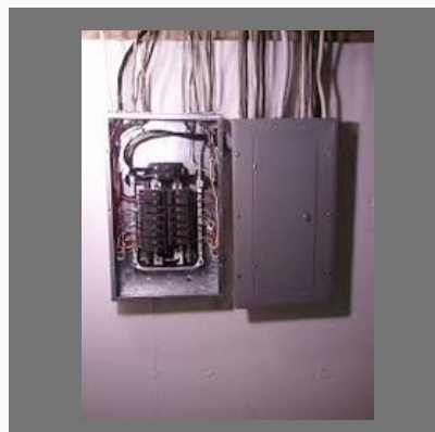
Installation of Electrical Gadgets
