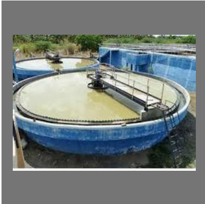
Water Supply And Sewage Treatment Plants
