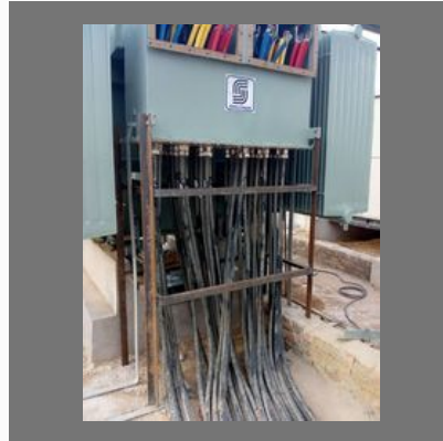
HT LT Switchgear Retrofitting
