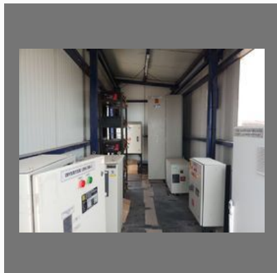
Roof Solar Power Plant Installation
