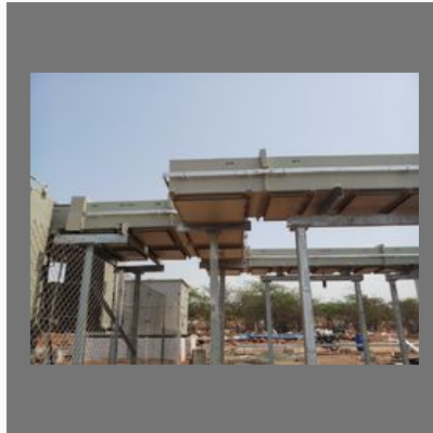
MS Fabrication Service For Bank
