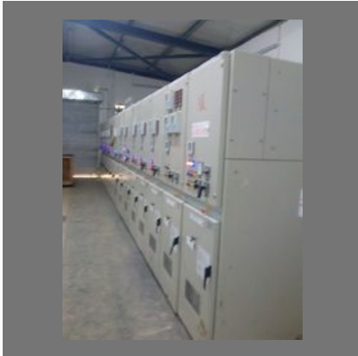
Solar Power Plant Installation
