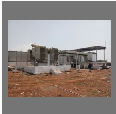
MS Fabrication Service For Bank
