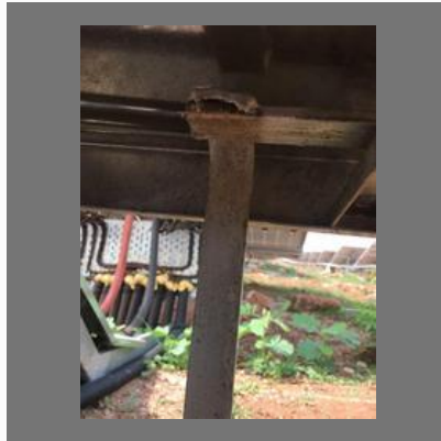
MS Fabrication Service For Bank
