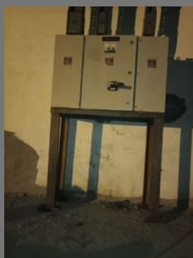
Off Grid Solar Installation Service
