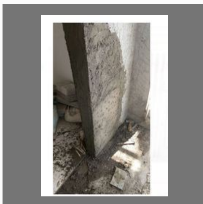
Wall Construction Work
