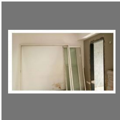
Bedroom Construction Service
