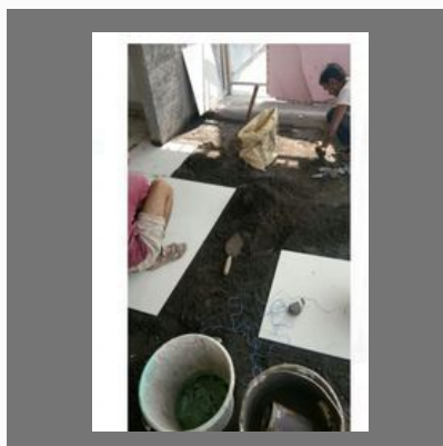
Kitchen Construction Work
