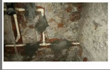
Bathroom Pipe Fitting Service
