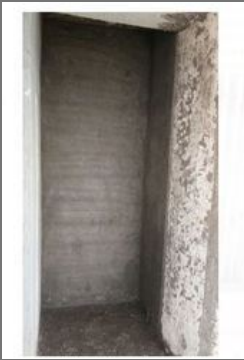
Bath Construction Work
