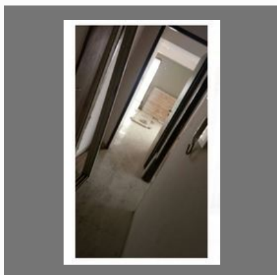
Kitchen Construction Work
