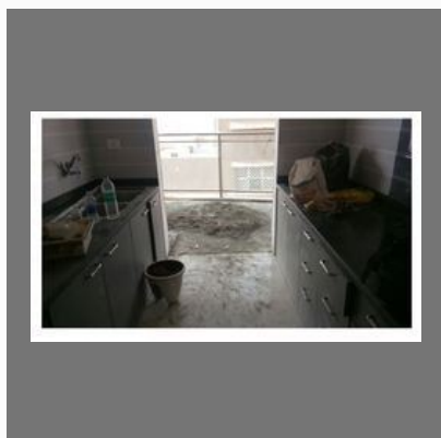
Kitchen Construction Work
