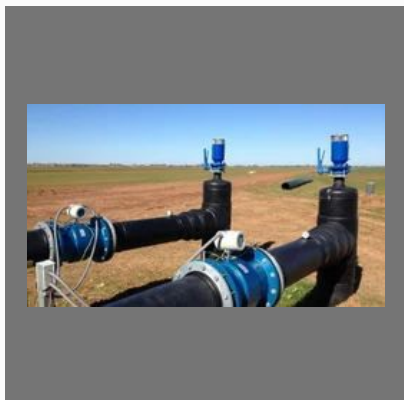
Water Flow Meter Installation Service
