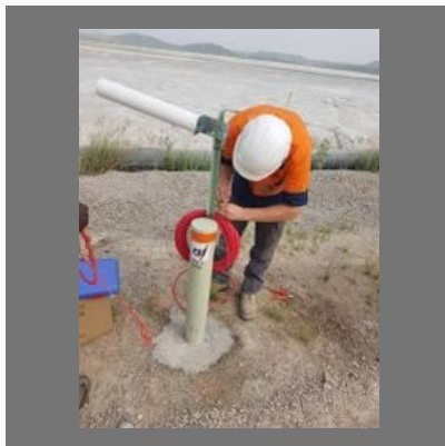
Piezometer Installation Service
