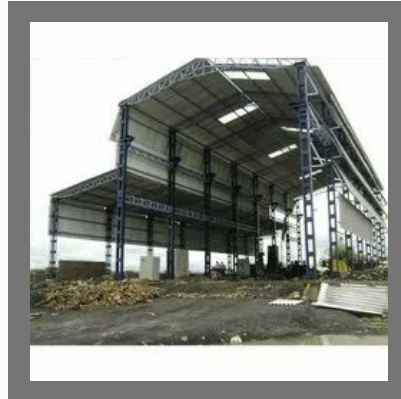
Industrial Shed Fabrication Works
