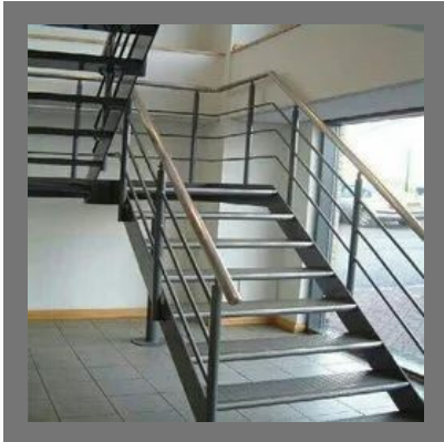
Mild Steel Staircase
