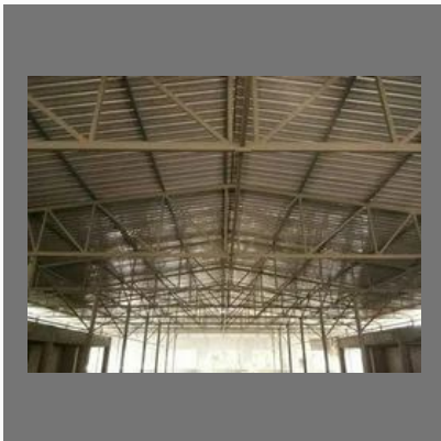
MS Fabrication Shed
