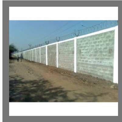
Compound Boundary Wall
