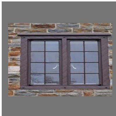
Steel Window Frame
