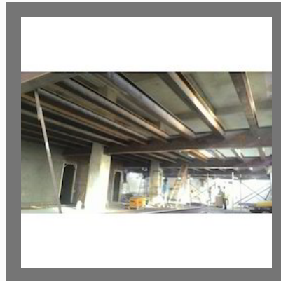
Structural Fabrication Service
