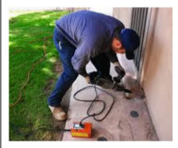
Post-Construction Termite-Proofing
