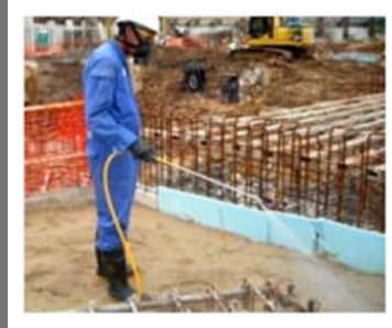
Pre-Construction Termite-Proofing
