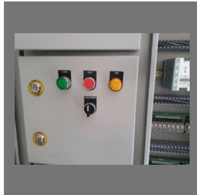
Servo Voltage Control Panel
