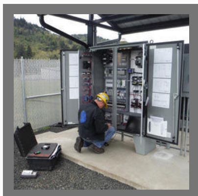
Control Panel Repairing Service
