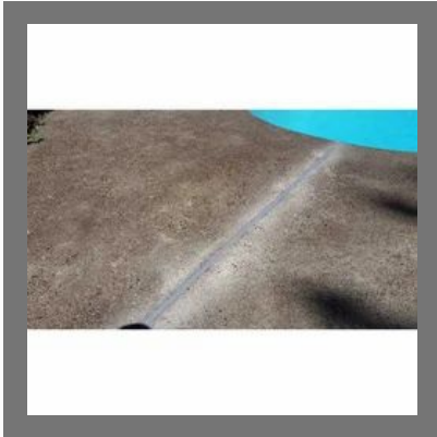
Epoxy Expansion Joint Sealant Filling Service
