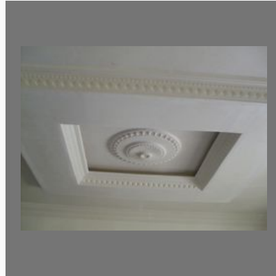
POP Ceiling Work
