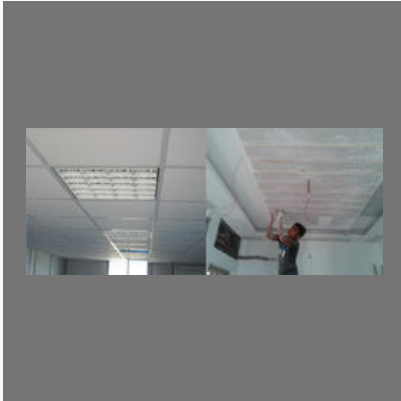
Gypsum Ceiling Work
