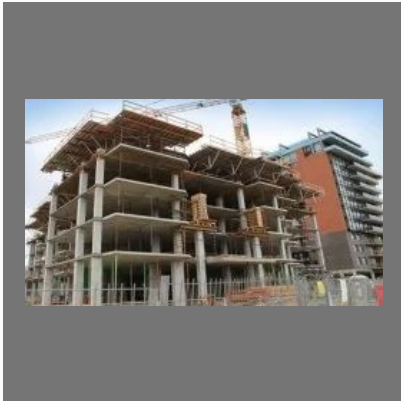
Residential Building Construction
