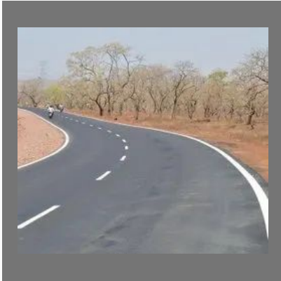
Highway Bitumen Road Construction Services
