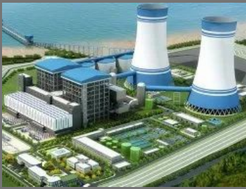
Thermal Power Plant Construction
