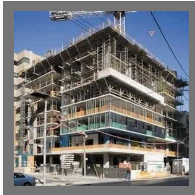
Construction Of Administrative Building
