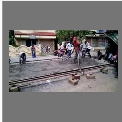
Concrete Road Construction Service
