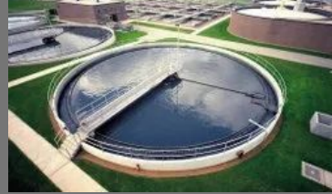
Effluent Treatment Plant Construction
