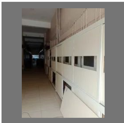
Aluminum Window Section Fabrication Work
