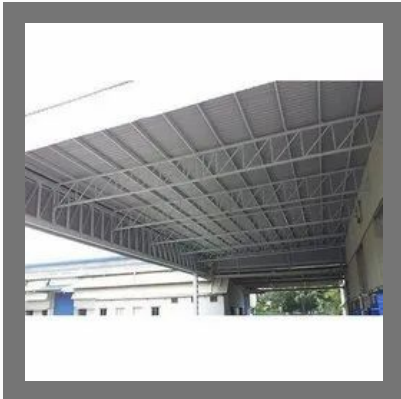
Roof Structural Fabrication Service
