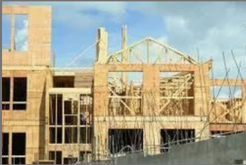
Commercial Building Construction
