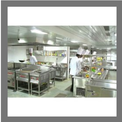
Commercial Restaurants Kitchen Equipment Consultancy Services
