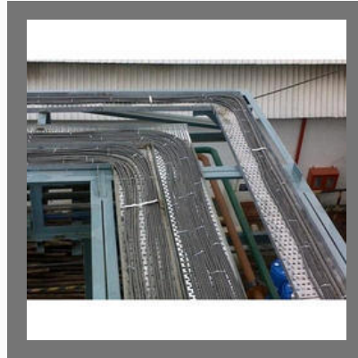
HT Cable Laying Services
