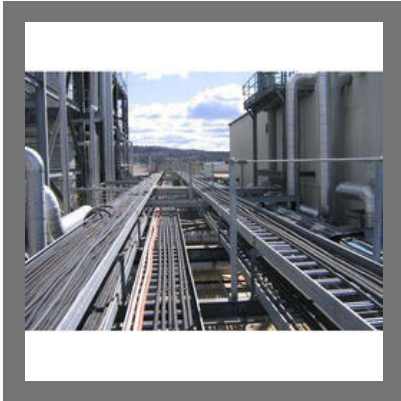
Cable Laying Services
