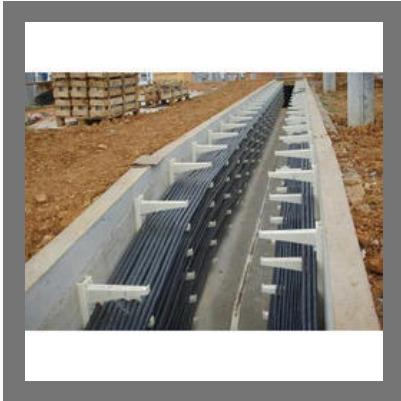
LT Cable Laying Service
