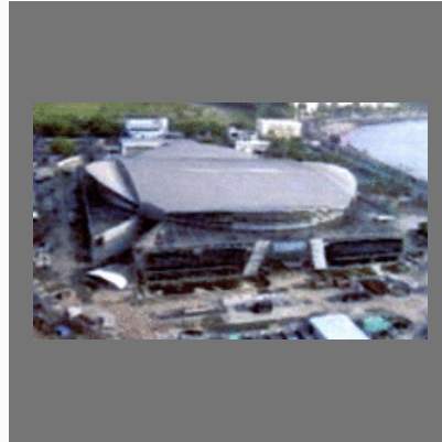
Steel Fabrication Works
