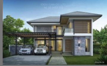
2 Story House Construction Service
