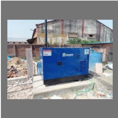
15 Kva Silent Diesel Generator Set
