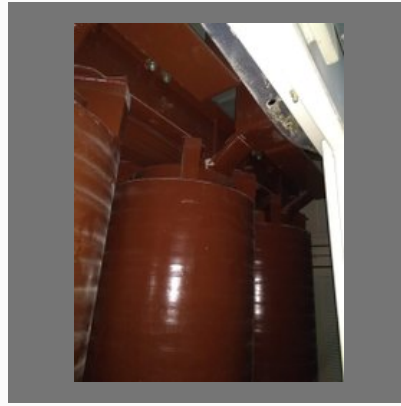
1 Phase Of 2,000 Kva Dry Type Transformer Changed Along With Servicing
